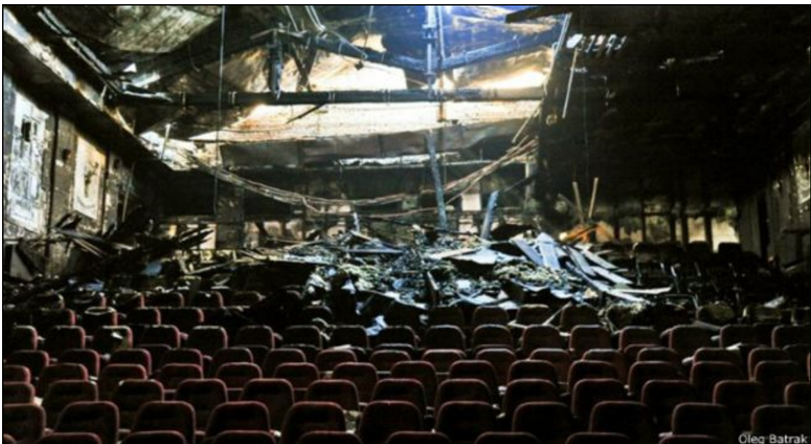
The screening hall ruined as a result of the arson.
